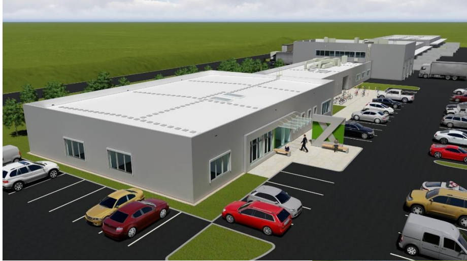
Technical building extension (2021)
